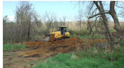
Building a trail crossing at Pierce Creek Park.
